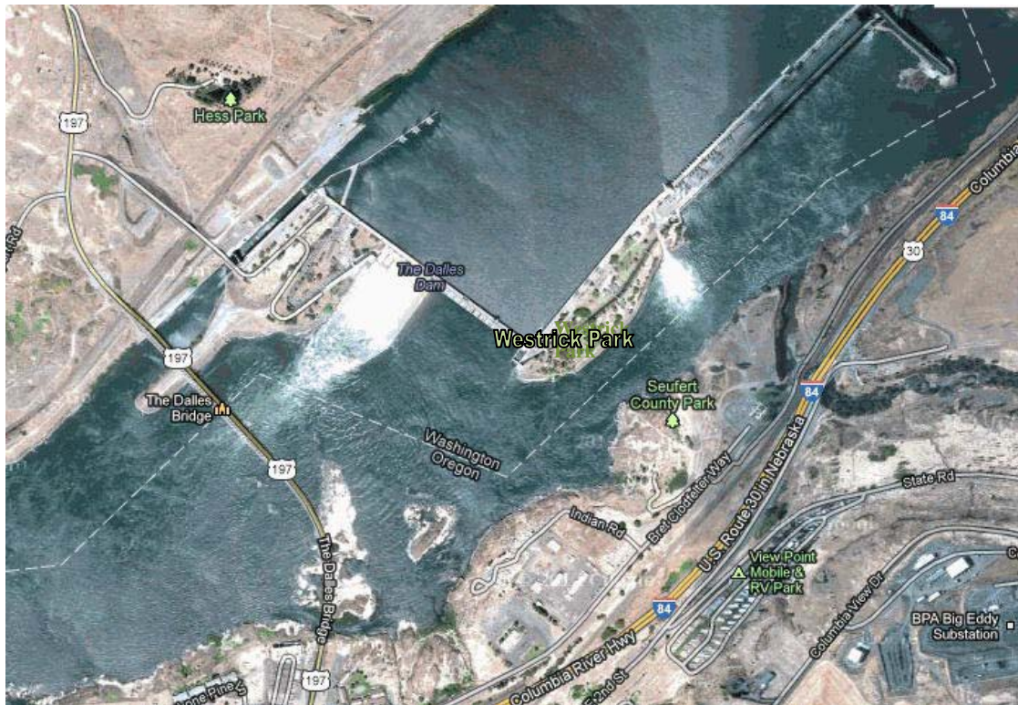
Figure 1. Image of The Dalles Dam April 2012 from Google© maps.
